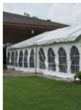
Installation of Tent Sides | $75
