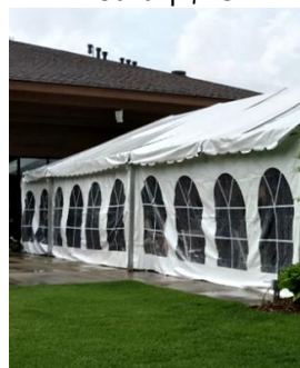
Installation of Tent Sides | $150
